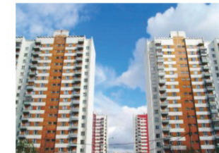
▲ Residence in Brazil Specs: 12 units Elevators
