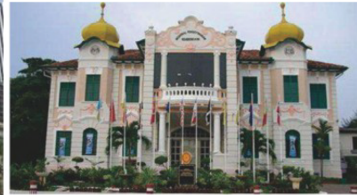
▲ Location: Sudan Project Name: Government Building
