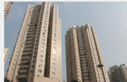
▼ Residence in India Specs: 18 units Elevators
