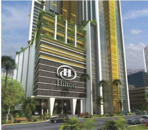
◀ Location: Panama Project Name: Hilton Hotel
